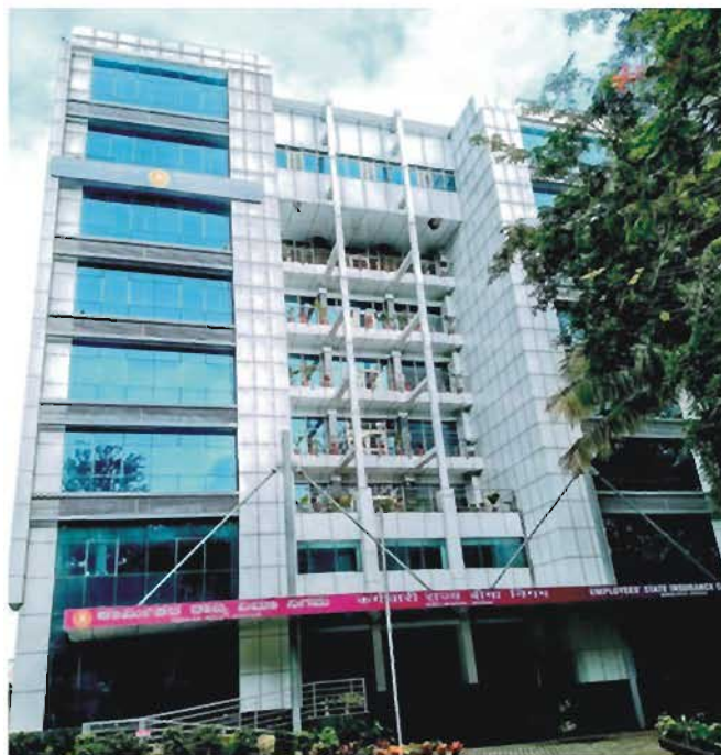
Regional Office, Bangalore – Nerve Centre of ESIC Operations In Karnataka
