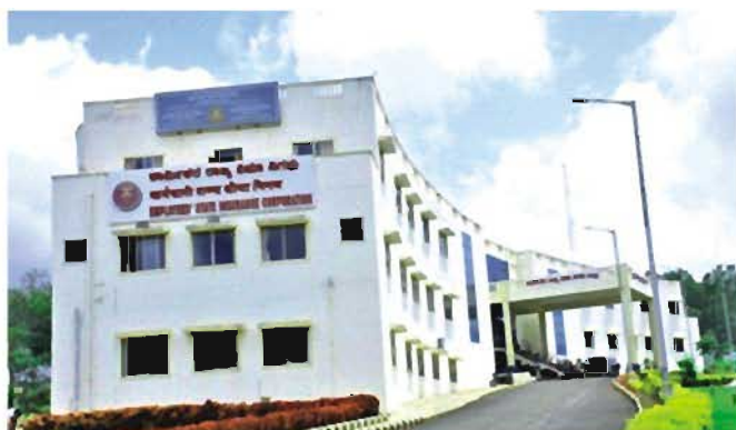
Newly Constructed Building of Sub Regional Office, Hubli, Karnataka
